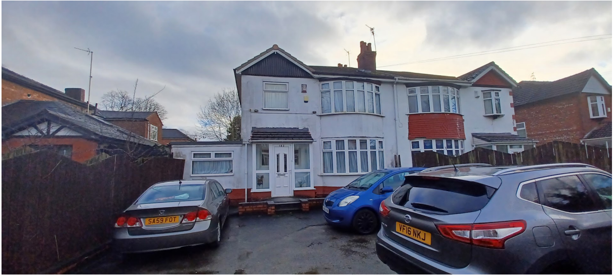
Figure 3. Principal elevation of property.
