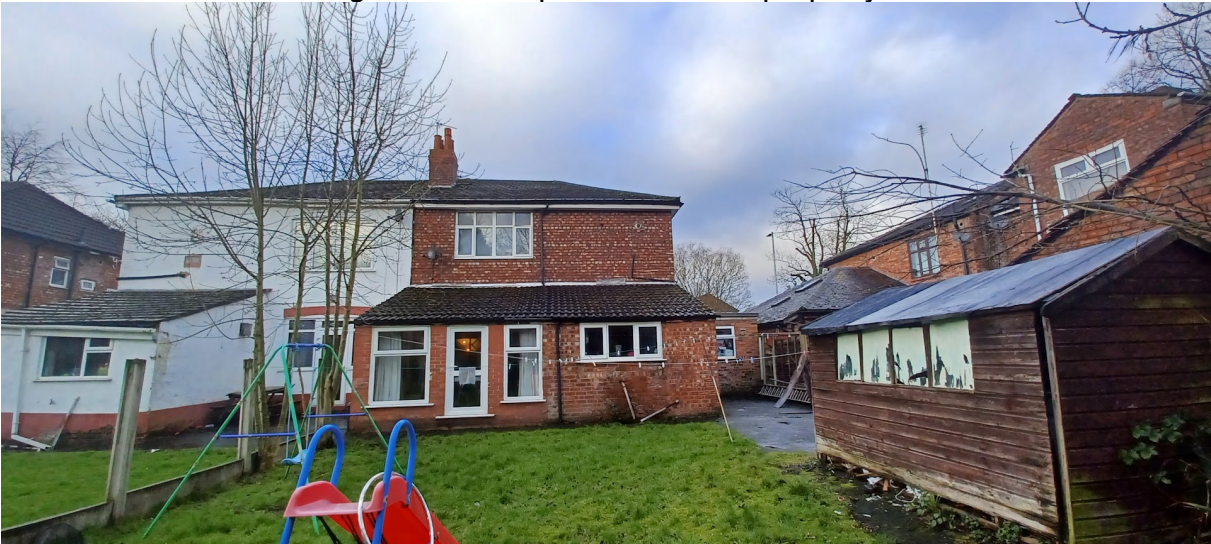
Figure 4. Rear elevation of property.
